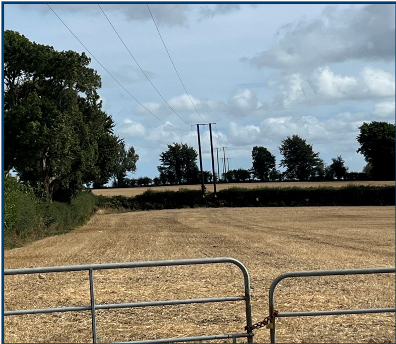
* Typical 38 kV Double Pole (longer span technology)
